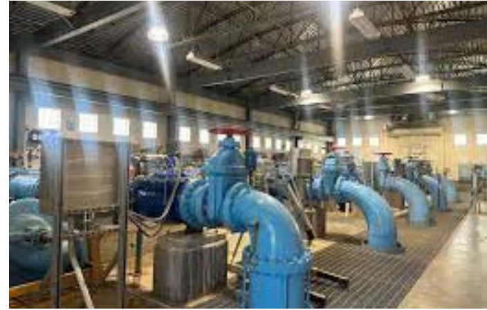
Figure #. West Travis County PUA Facility
